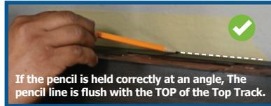
If the pencil is held correctly at an angle, The pencil line is flush with the TOP of the Top Track.
