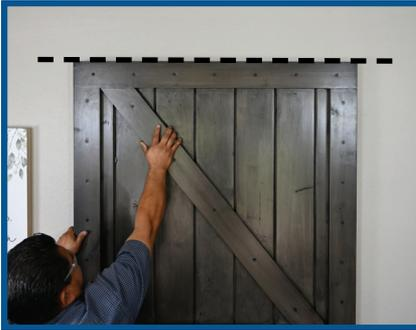
To determine the Wall Mount's vertical position, raise and position the door parallel to the wall (as seen in the image to the left). Once in position, **use a pencil to mark the top of the Top Track**, not the top of the door. This measurement is your vertical position.
