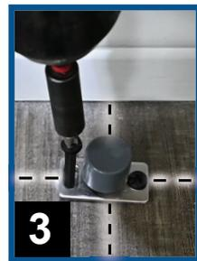
After using a pencil to mark the Door Floor Guide holes, use a drill to make two holes. Next, insert the (2) anchors in to the holes. Use the provided screws to firmly attach the Door Floor Guide. **Do Not Over-Tighten.**
