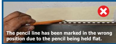
The pencil line has been marked in the wrong position due to the pencil being held flat.
