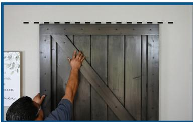
To figure out exactly how high the Wall Mount should be installed on the wall, lift the Door Slab up and position as closely as you can to the wall. This step may require two people to perform. See page 14 for further information.
