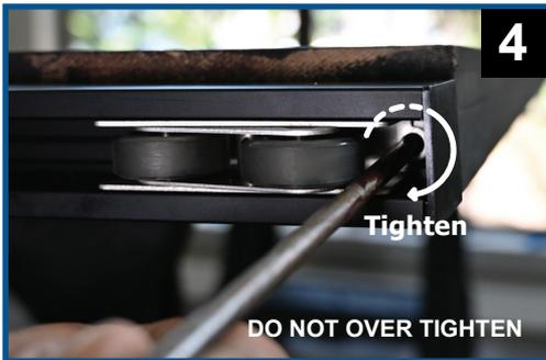
Make certain that the Bottom Track is moved forward to be completely FLUSH with the front side of the door before installation (as shown in the image to the right).
